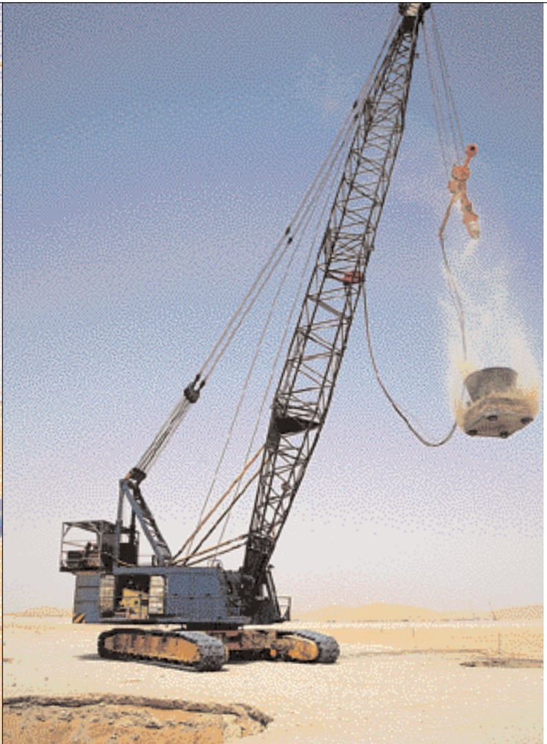
THE MARS PROCESS (MENARD AUTOMATIC RELEASE SYSTEM) optimizes the energy from ground compaction by eliminating energy loss from braking or friction.
