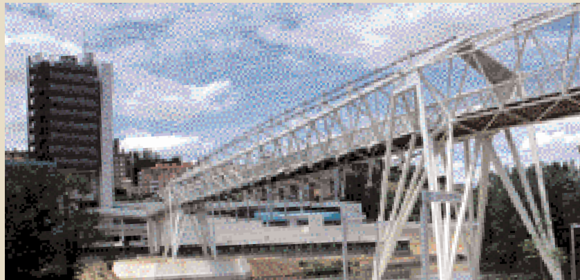
The cables of the Valladolid Science Museum footbridge serve both as stay cables and prestressing elements.
