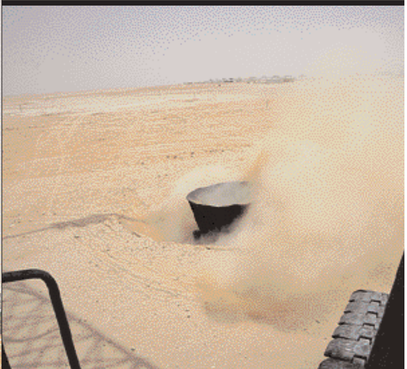
THE MARS PROCESS (MENARD AUTOMATIC RELEASE SYSTEM) optimizes the energy from ground compaction by eliminating energy loss from braking or friction.
